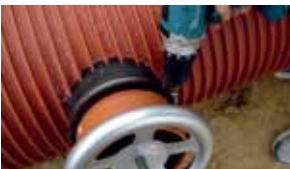
Before removing the tool tighten the tightening strap with 8Nm.
