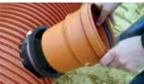
Insert the pipe into the Insitu Seal.
