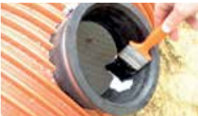
Coat the inside of the seal with lubricant (not under the clamp band).
