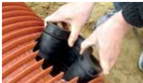
Position the Insitu Seal into the drilled hole until the collar reaches the inside of the pipe.
