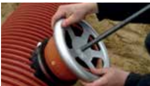
Use the assembly tool to position the seal correctly.
