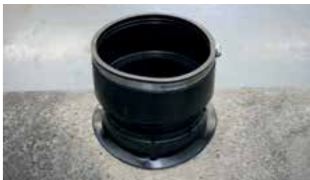
Place the element flush, observe the radius.
