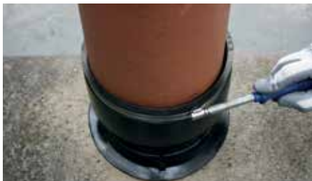
Tighten the tensioning strap with 6 Nm.
