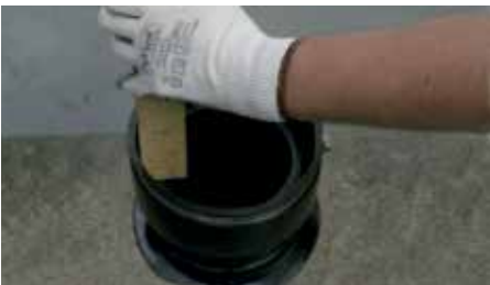
Drive in the clamping sleeve flush with the driving-in aid.
