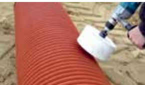
Drill a hole in the specified size and deburr the hole.
