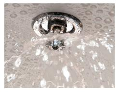
Unique air pressure monitoring takes readings 2x per second to automatically adjust to both small and slow changes in system air pressure, but trips when there is a steady drop in system air pressure upon sprinkler operation.
