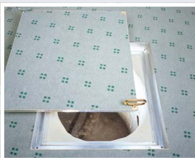
BVA installed in an office (over a manhole), in a carpeted area
