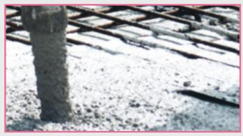
For this reason we recommend using a type of concrete that, when fresh, has high fluidity without causing segregation phenomena in the components (fig. 3).
