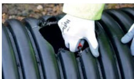
Remove any burring or flashing from the edges of the hole.
