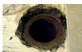
flush cut pipe
