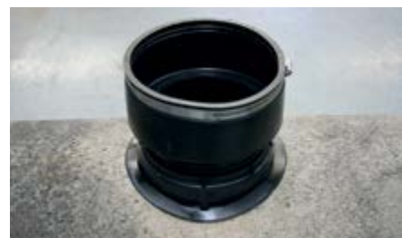
Place the element flush, observe the radius.
