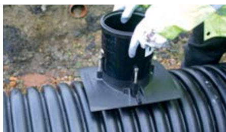
Insert the adaptor, as received, into the hole so that the saddle flange sits snugly onto the pipe OD.
