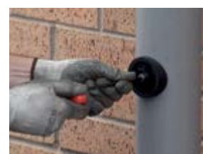
tighten the fastener
