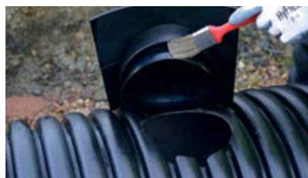
Apply lubricant to the outer face of the inner sleeve and seal in the area.
