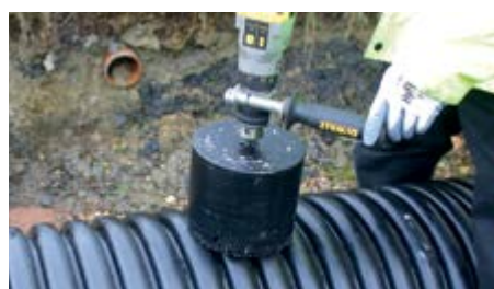
Drill a core hole with 177 mm (+ 2mm / -0.5 mm) diameter.
