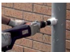
drill a core hole
