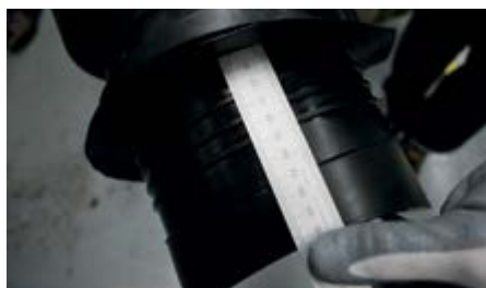
Adjust the screw collar according to the wall thickness.
