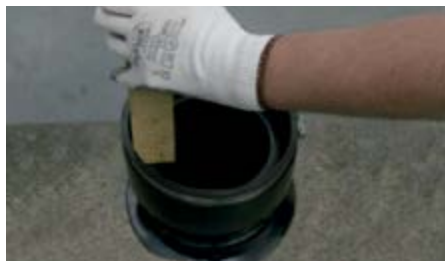
Drive in the clamping sleeve flush with the Impact Aid.
