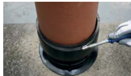
Tighten the tensioning strap with 6 Nm.
