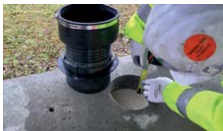
Make a core hole and deburr the hole.
