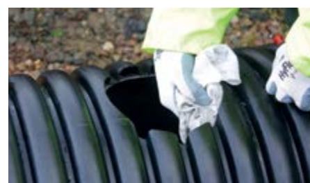
Wipe the inside surface clean.
