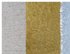
Example: Aerated concrete, mineral wool, plaster
