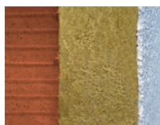
Example: Perforated brick, mineral wool, plaster
