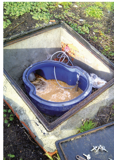
Example of a grease separator needing to be emptied
