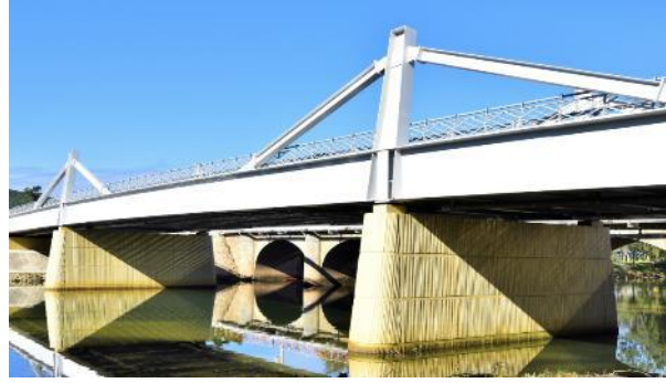
Dumbea Bridge - Noumea - New Caledonia Itinero®
