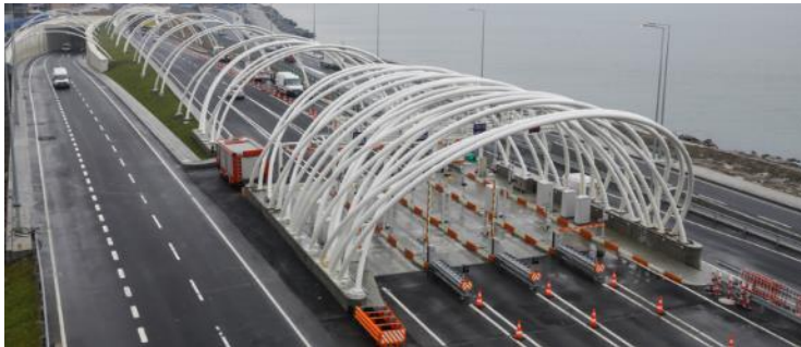
Eurasia Tunnel - Istanbul - Turkey S range
