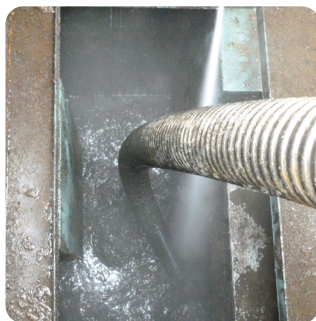
Cleaning the walls with high-pressure jet
