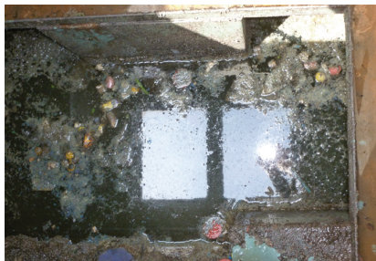
View of sludge trap chamber
